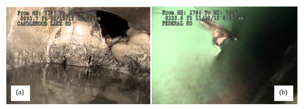
Figure 3-7 (a) Grease at downstream end of 2797-2799. (b) Intruding Object through Pipe Wall of 2784-2802 at 234 LF from upstream manhole.
