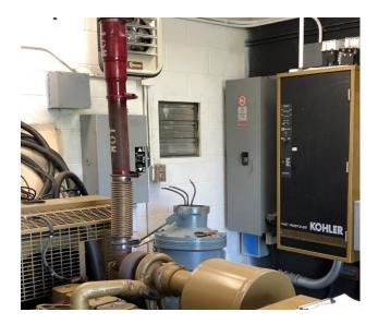
• The TVSS surge protector lights are currently not working. This could indicate the equipment is no operating correctly and not providing adequate protection to the pump station from power surges. We recommend to replace the TVSS surge protector.
