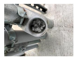
• The vent pipe is located 4'-10" from the generator. It is recommended to rotate the vent pipe to face the opposite direction of the generator to provide a 5'-0" clearance.
